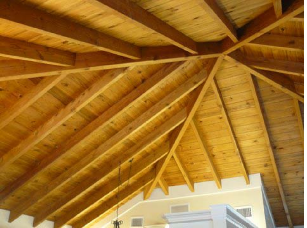
Original cypress ceilings were preserved
