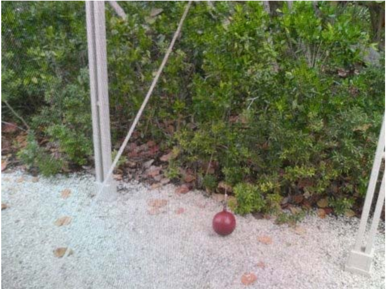
Photo Caption: Often referred to as the “Cannonball House,” the Walker guest house was designed by Paul Rudolph with walls that open the interior to nature by a series of pulleys and weights in the form of large red balls.
