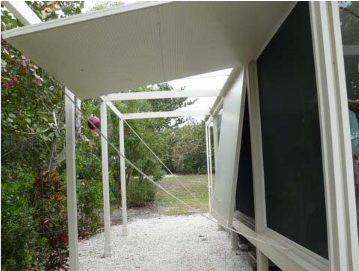
Photo Caption: Weighty red balls hold the “flats” or walls up making nature an integral part of the Walker guest house experience.
